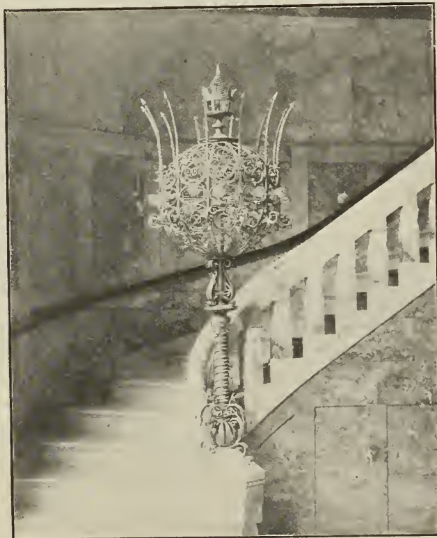
B.—ELECTROLIER AND NEWEL. Mills Building, San Francisco, Cal. Wrought Iron, Hammered Leaf, Bower-Barffed.
